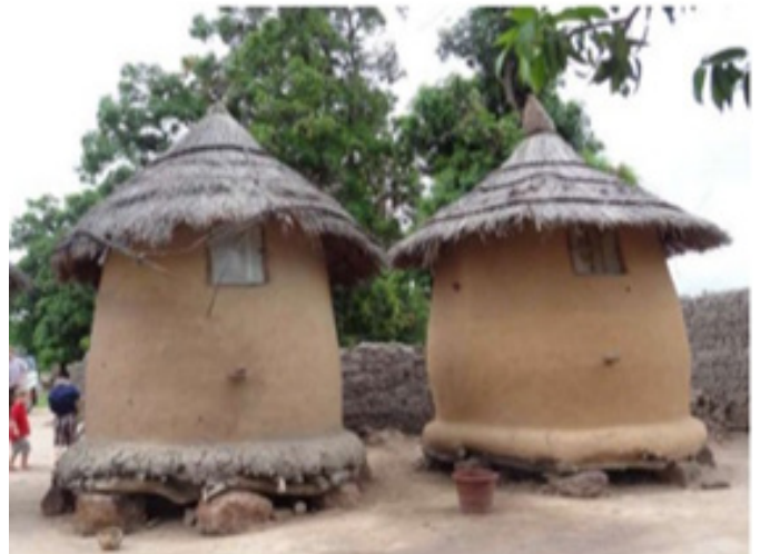
Local storage system
